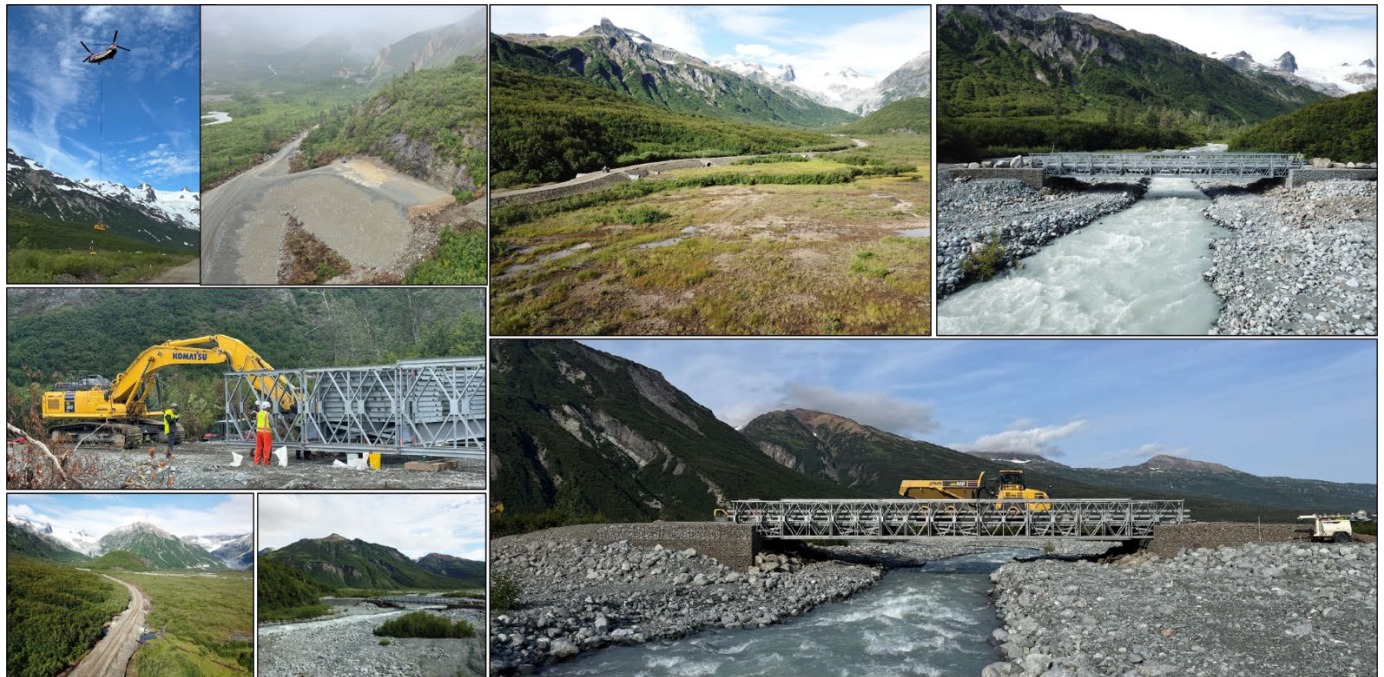
FIGURE 2: Construction progress and development of the road from camp to the proposed portal location with two bridge crossings at Double Glacier Creek and Johnson River.
