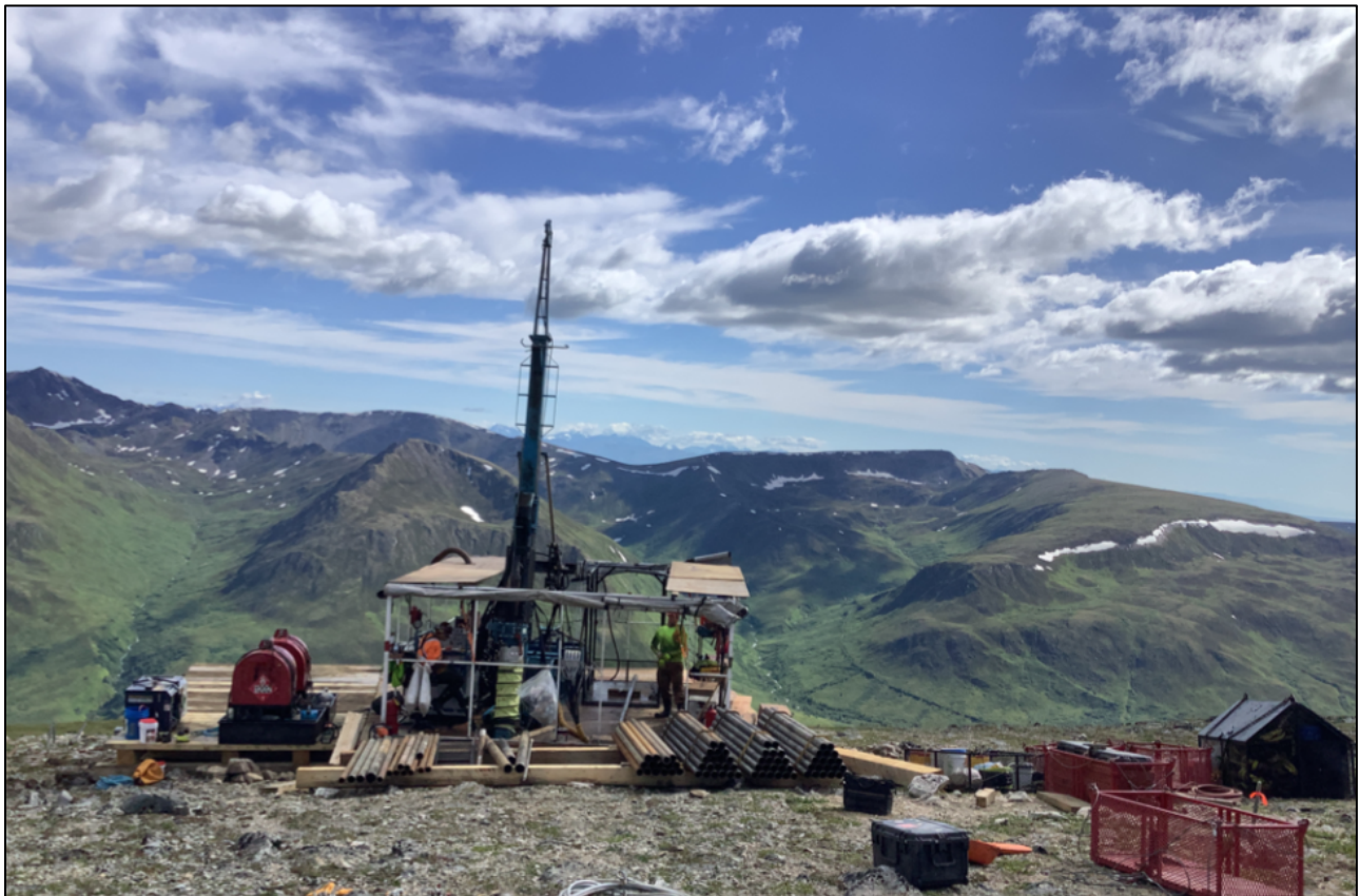
Figure 1. Helicopter-supported diamond core drill operating from Coleman Pad D on Lucky Shot Ridge.
