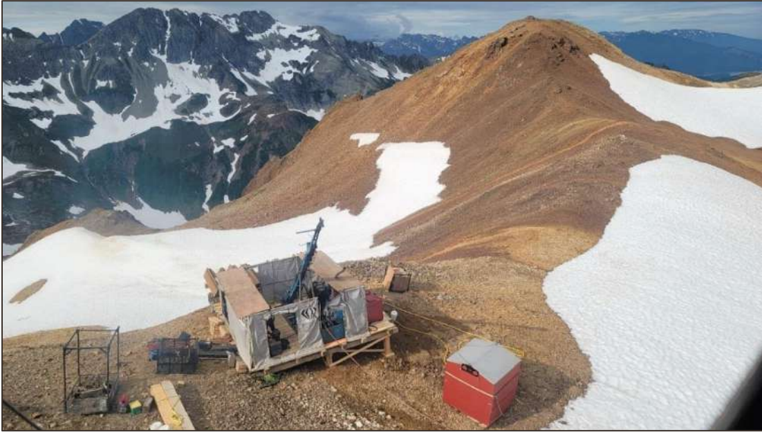
Plate 10.1 Hy-Tech's TECH5000 Drill Rig at Upper Difficult Creek
